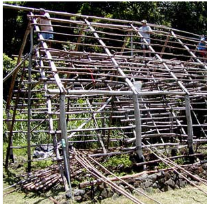
Hale Kutai under construction on Maui
